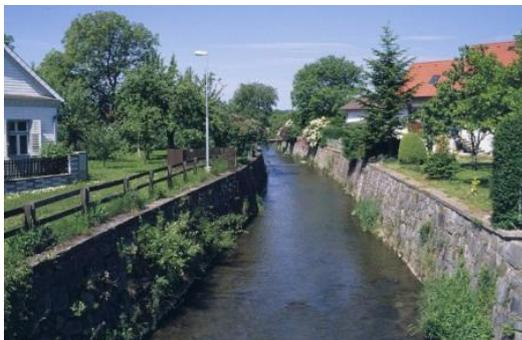
**Figure 22: stone pitching tightly packed**
