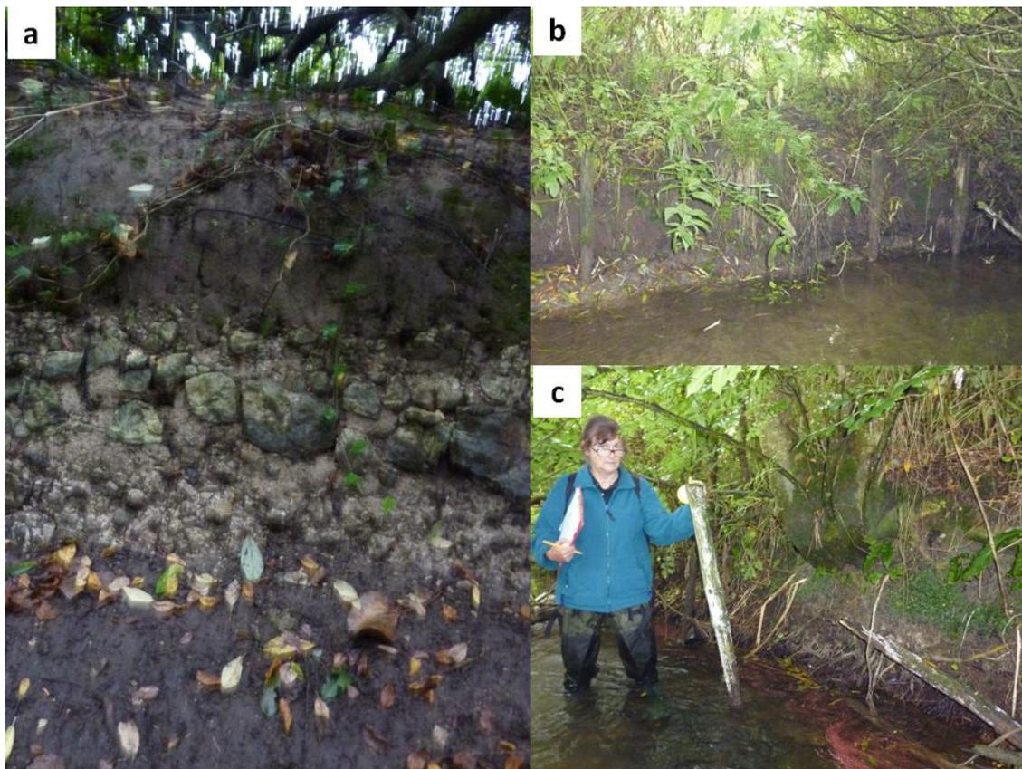
**Figure 8.11 Exposures of old bank reinforcement: a) stones, b) wooden stakes facing the bank, c) wooden stakes exposed by bank erosion and retreat.**
