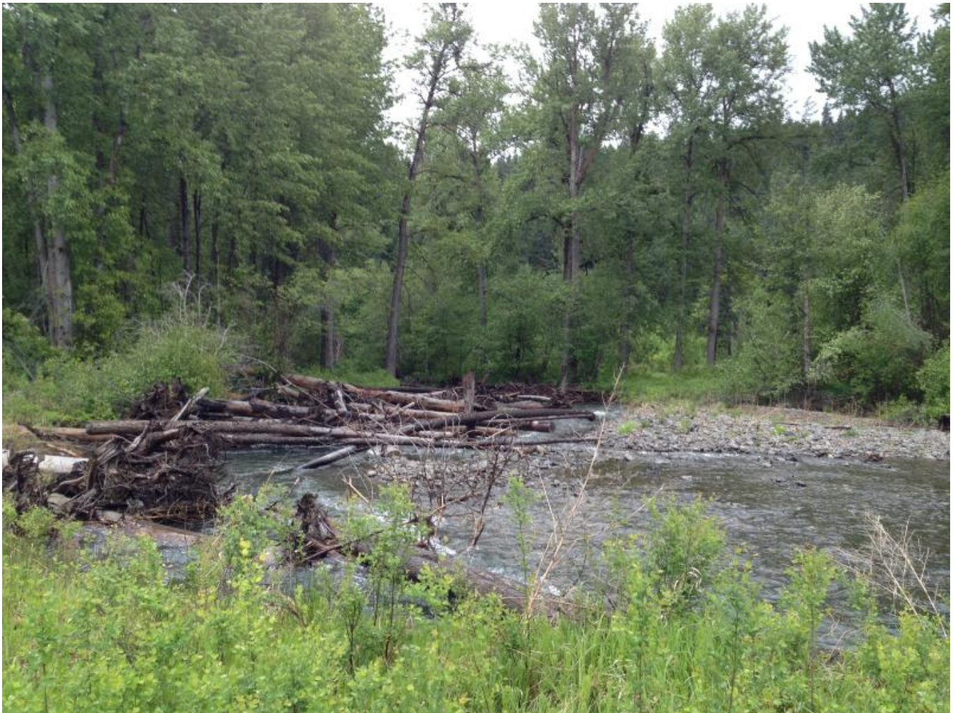
Photo: Placed logs in a stream to help restore in-channel habitat and reconnect floodplain wetlands in Washington State (photographer: Phil Roni)
