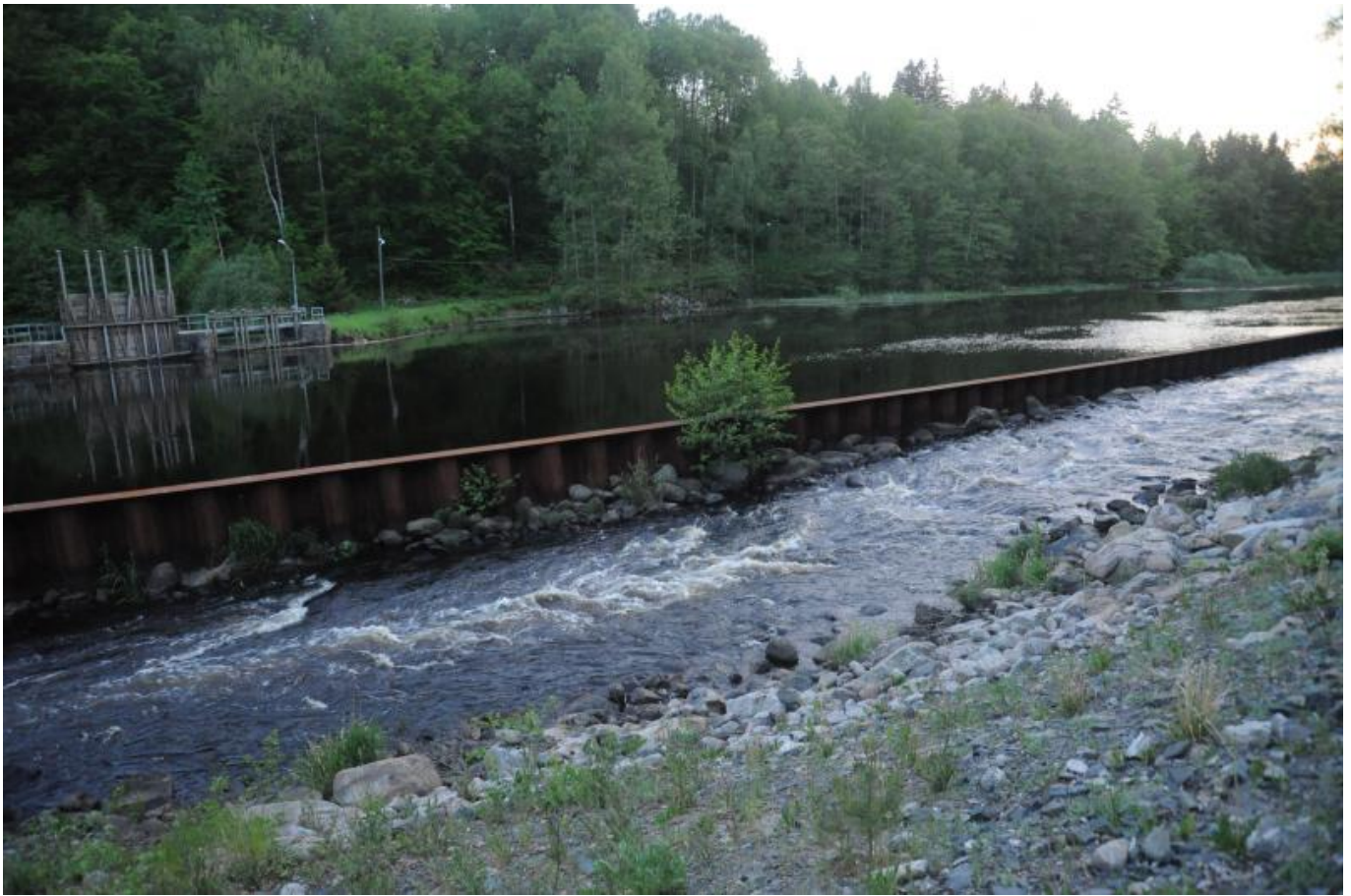
Figure 2. Nature-like partial width rock ramp constructed at Hemsjö nedre hydropower dam in River Mörrumsån in 2003-2004. Photo by Frauke Ecke, SLU.
