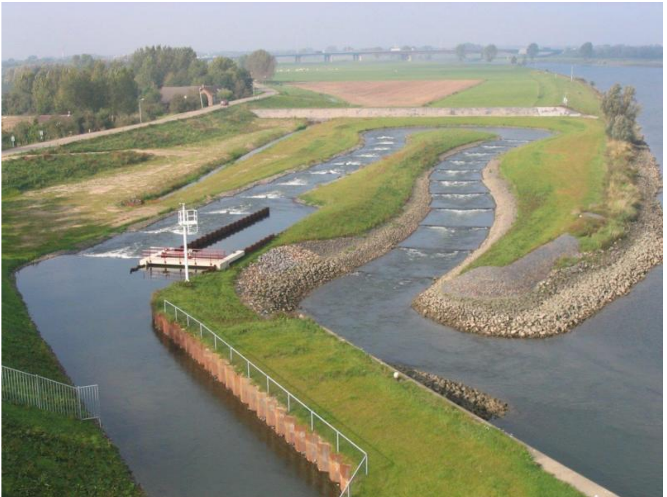
Figure 1: Fish passage at the weir Hagestein, location: River Rhine (more precisely the Rhine branch named 'Lek') near Hagestein, the Netherlands, 13 October 2004 (photographer: Tom Buijse)
