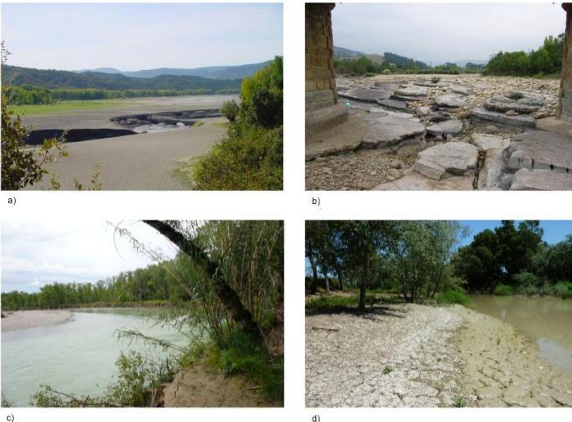
Figure 2.- a) Reservoirs are sediment traps. Barasona Reservoir in R. Esera (Ebro Basin). Over 80 % of reservoir capacity has been lost. b) Armouring river bed (R. Pas). Incision caused by smaller substrate size selective erosion. c) Lateral bank erosion in meander. R. Gallego. d) Sediment deposits in lateral banks. R. Guadalete (photo by D.G.De Jalon, 2015)
