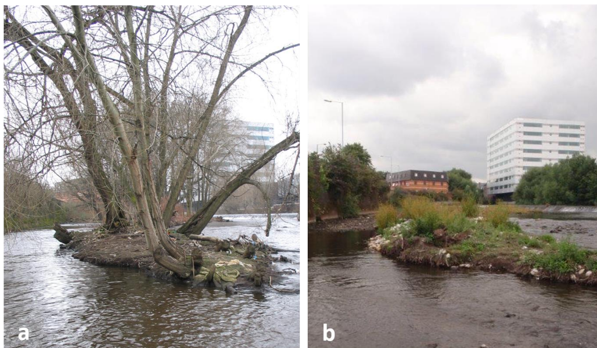
Figure 2.5. Removal of trees to reduce the risk of flooding on the River Don a) before and b) after flood defence works (source: Jon Harvey).
