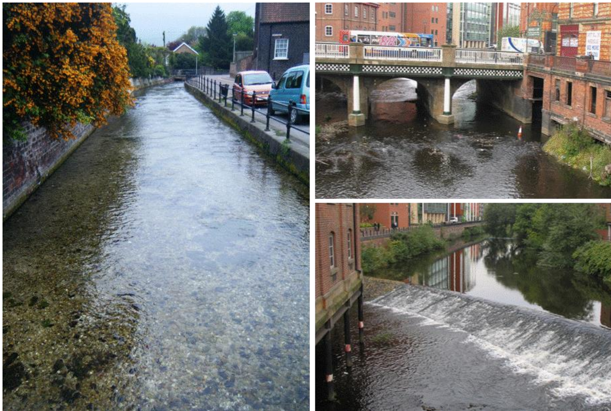
Figure 2.3. Urban rivers and streams showing many of the main urban pressures such as increased impervious surfaces, channelization, fragmentation, artificial river bed, reduced instream and bankside vegetation (source: Natalie Angelopoulos).
