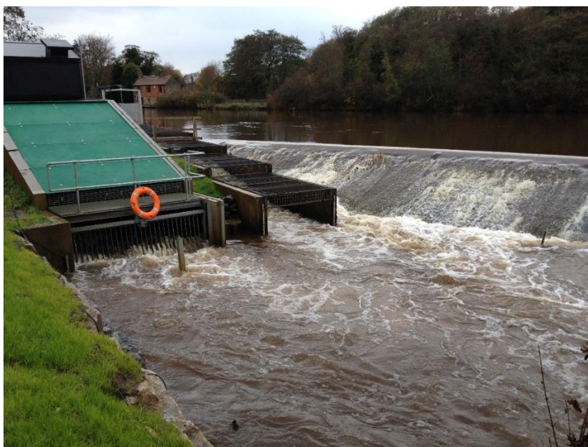
Figure 2.9. An example of how opportunities arise between hydropower scheme and the restoration of longitudinal connectivity to improve fish passage along an existing barrier. Hydropower on the left and a Larinier fish pass to the right (source: Jamie Dodd).
