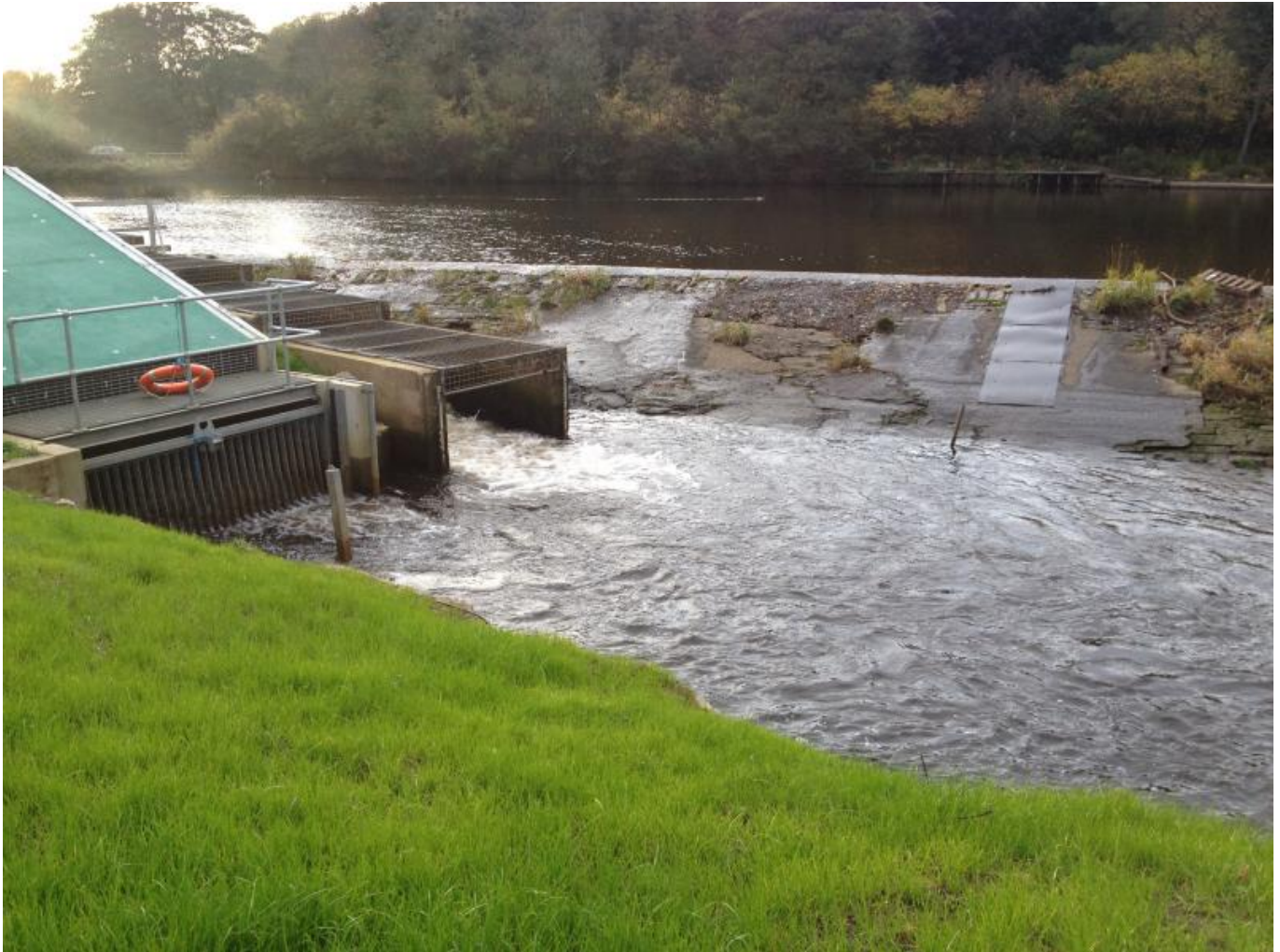
Figure 2: An example of how opportunities arise between hydropower scheme and the restoration of longitudinal connectivity to improve fish passage along an existing barrier. Hydropower on the left and a Larinier fish pass to the right (photo: Jamie Dodd).
