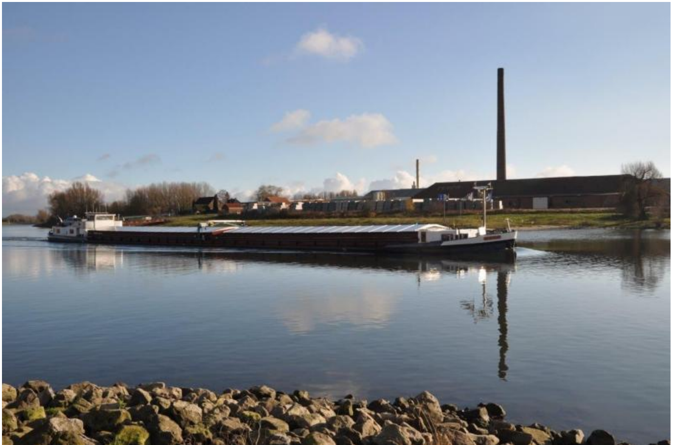
Figure 1: Riprap and groyne contribute to maintaining the navigable depth in rivers (photo: Tom Buijse)
